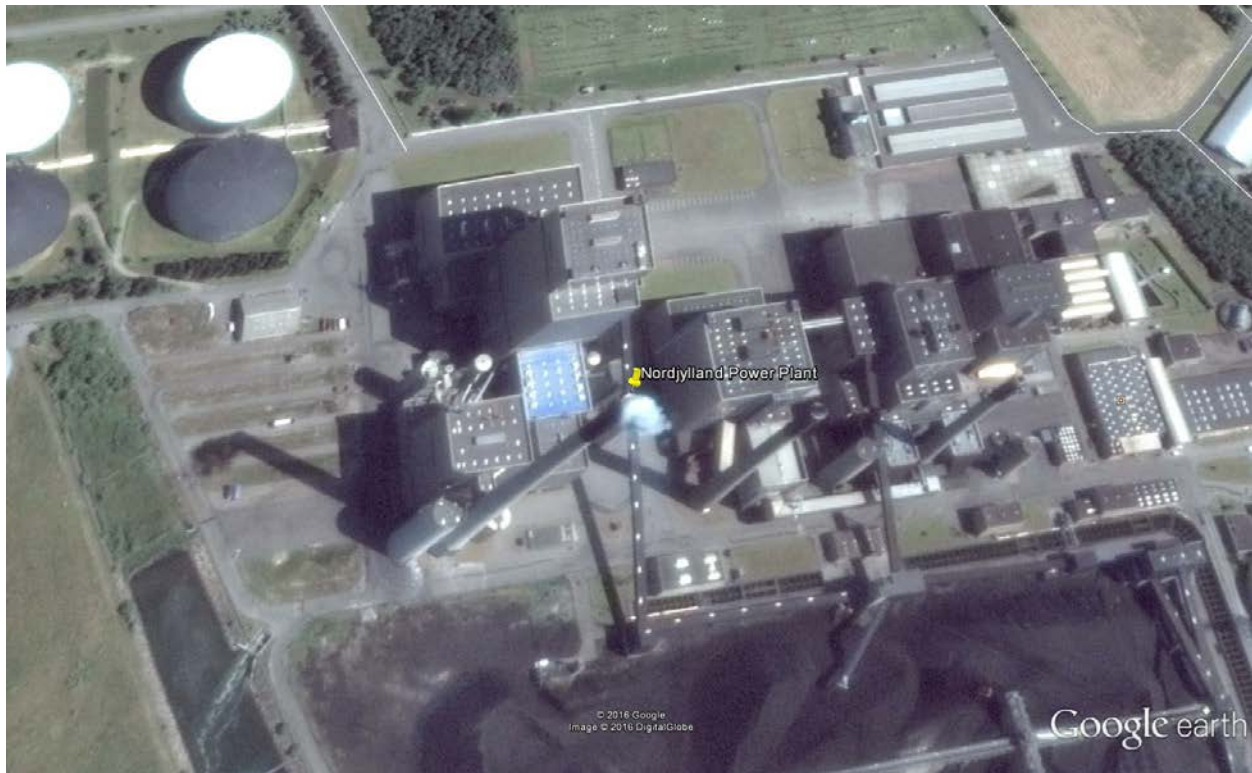
Figure 21. Nordjylland Power Plant, Denmark
