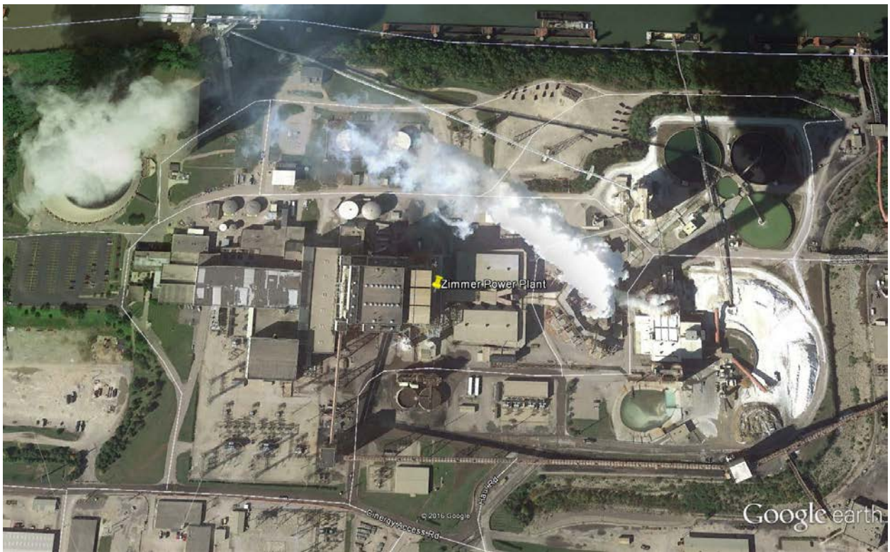
Figure 11. Dynegy's W. M. Zimmer Plant
