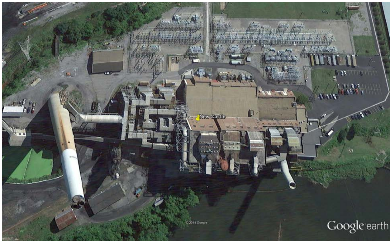
Figure 22. New Castle Power Plant
