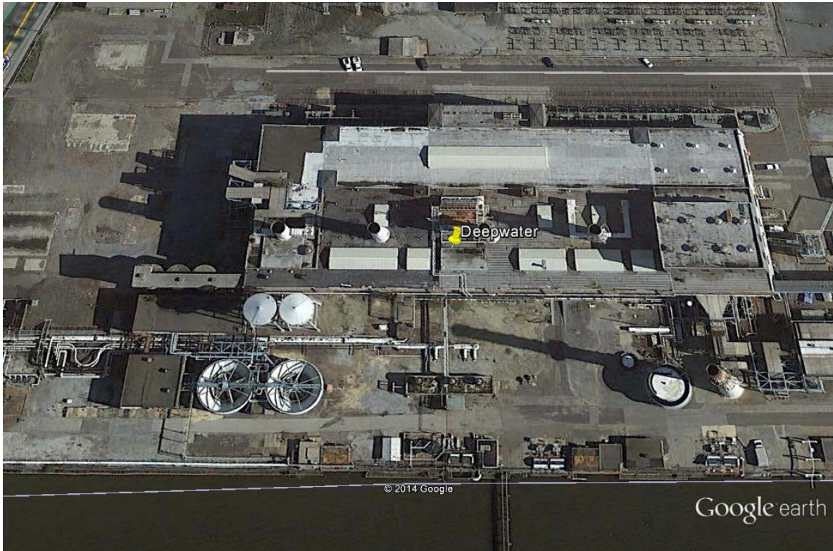
Figure 15. Deepwater Power Plant
