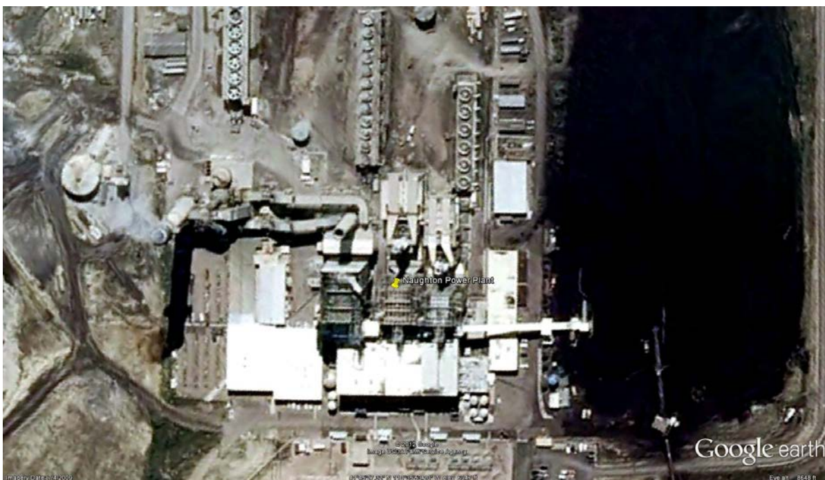
Figure 28. Naughton Power Plant
