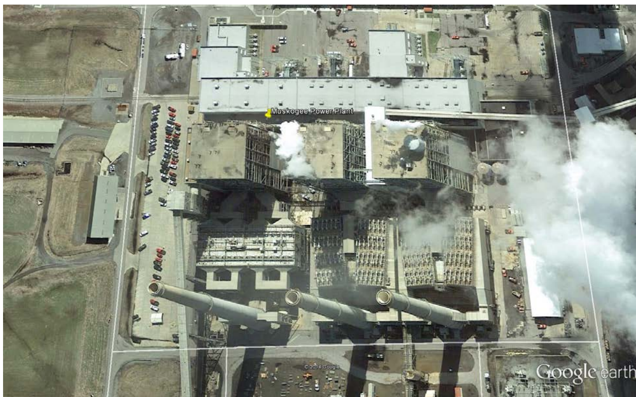
Figure 18. Muskogee power plant, units 4 & 5 are the two units to the right.
